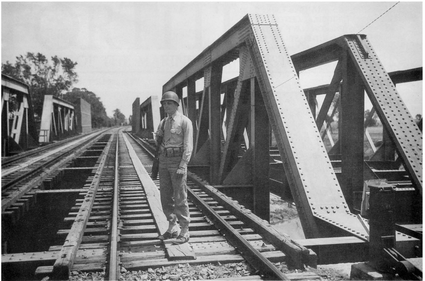
Marine Pvt William R. Deshler stands guard duty on Bridge No. 113 on the Peiping-Mukden Railway in May. Marine guards on the railways of North China helped to keep the highly populous
